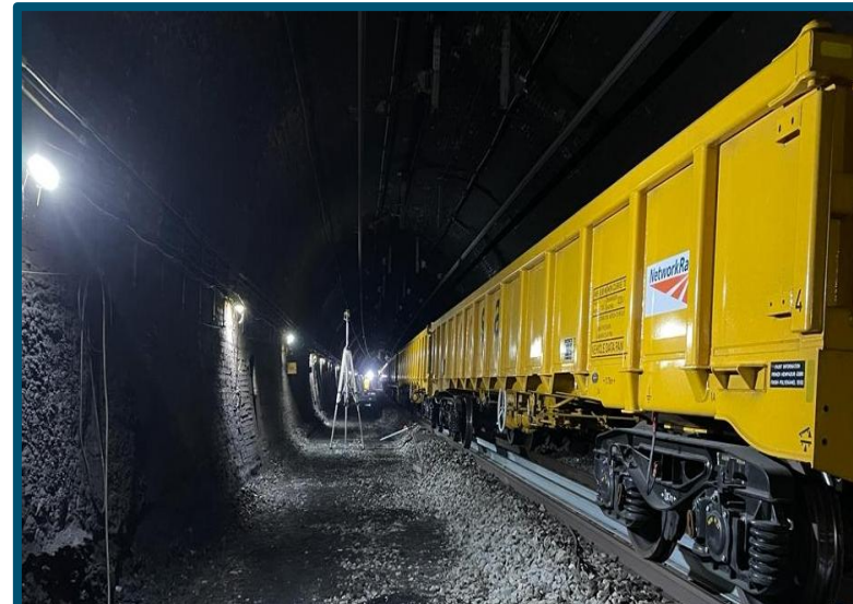
Work on the Severn Tunnel
