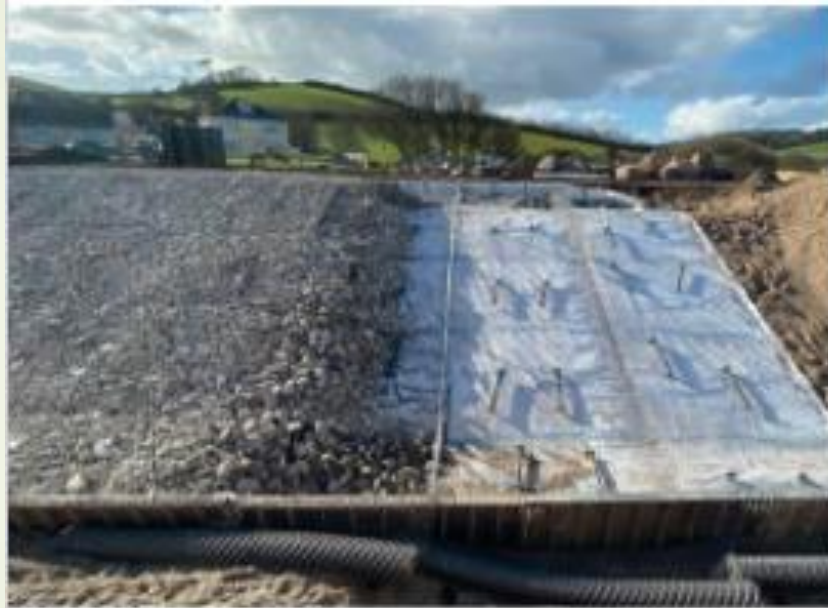
Tecco Cell: installation in 2021
