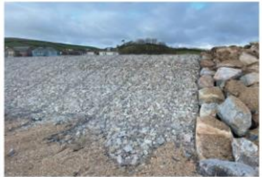
Finished installation of shore protection in 2021
