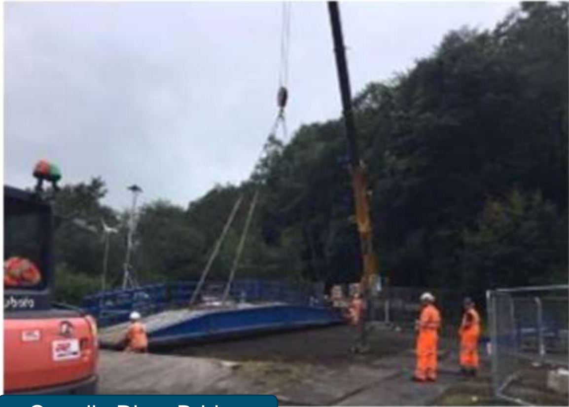
Crumlin River Bridge
