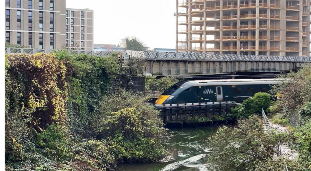
Voltage Clearance Control
